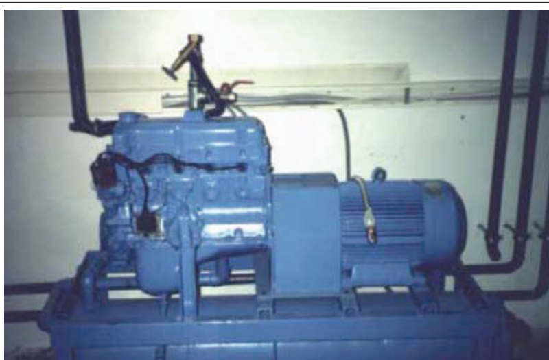
Figure 47: Co-generation unit (electricity and heat utilisation)
