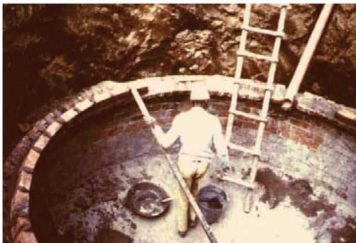
Figure 21: Construction of the weak/strong ring of a 16 m 3 , Tanzania Photo: Kellner (TBW)
