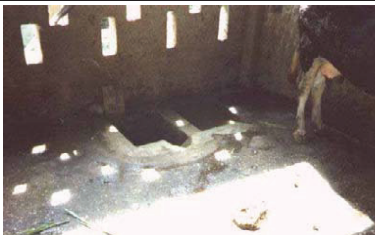
Figure 23: Cowshed, directly connected to the plant: A urine chamber to the right collects the liquid which can be used to wash the dung into the digester.
